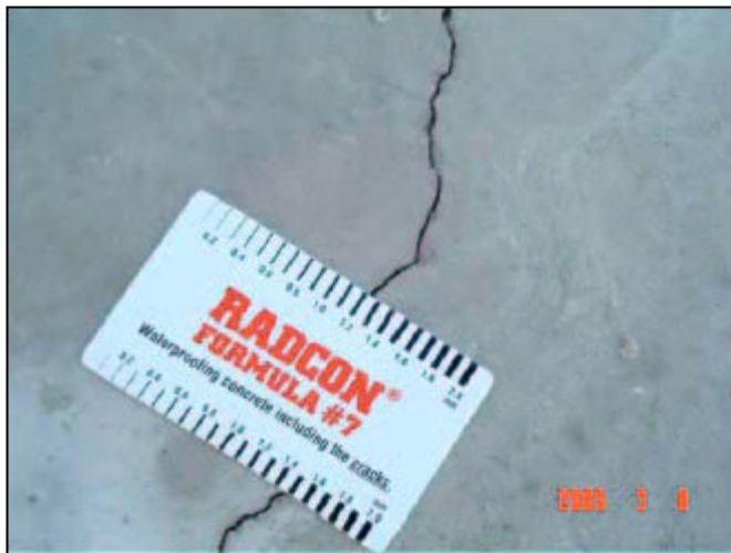
FIGURE 5 - 6 Existing cracks - 1.2 mm - Radcon Formula # 7 treated at a 1 litre / 5 linear meters rate before the application of the product at the remaining areas.
