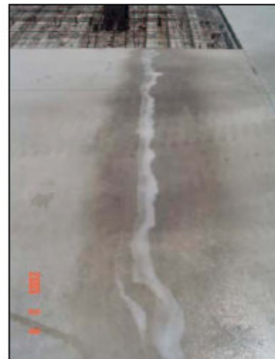
FIGURE 5 - 6 Existing cracks - 1.2 mm - Radcon Formula # 7 treated at a 1 litre / 5 linear meters rate before the application of the product at the remaining areas.
