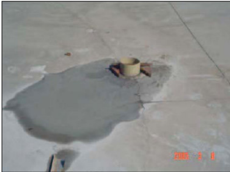
FIGURE 4. Drains and penetration treatment.
