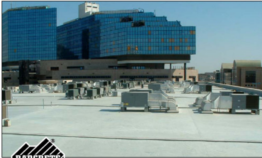
FIGURE 1. The first Radcon Formula #7 waterproofed rooftop of a shopping centre in Saudi Arabia
